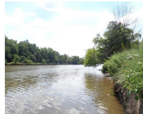
▲ Photo 10. View of existing seawall, looking north
