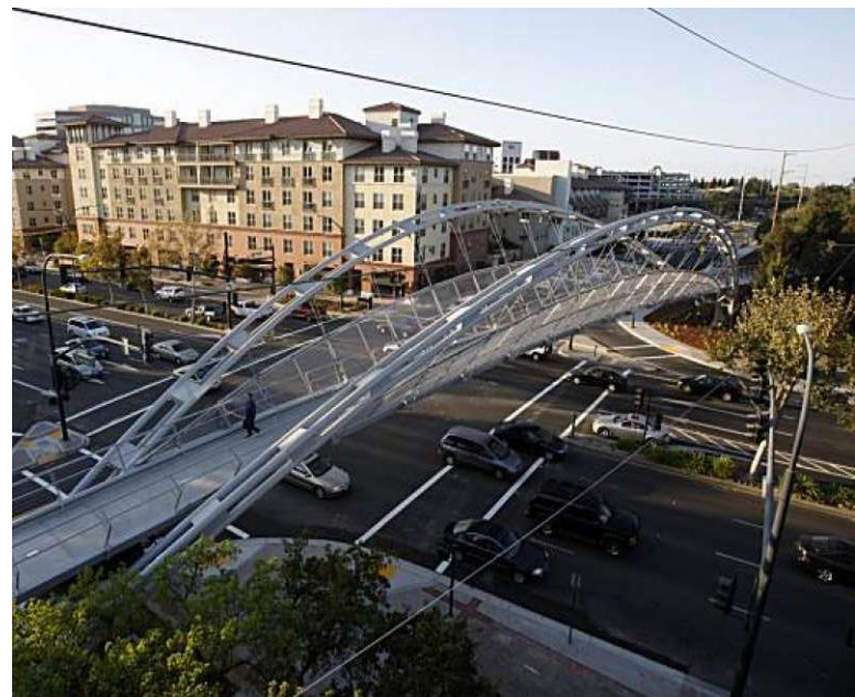
Schoder Overcrossing Contra Costa, CA 600 ft clear span pedestrian and cyclist bridge
