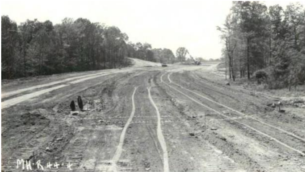
Final Construction- "B" Road
