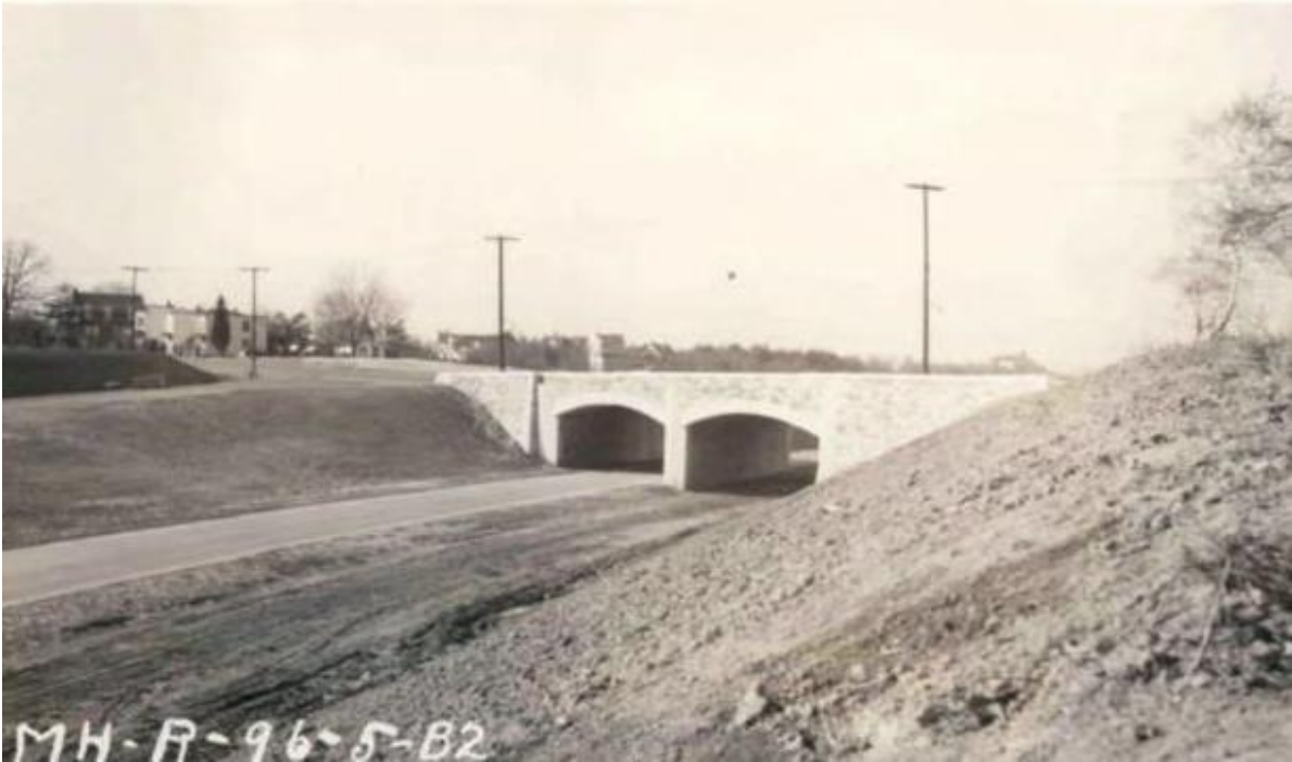
General view of east side of completed structure
