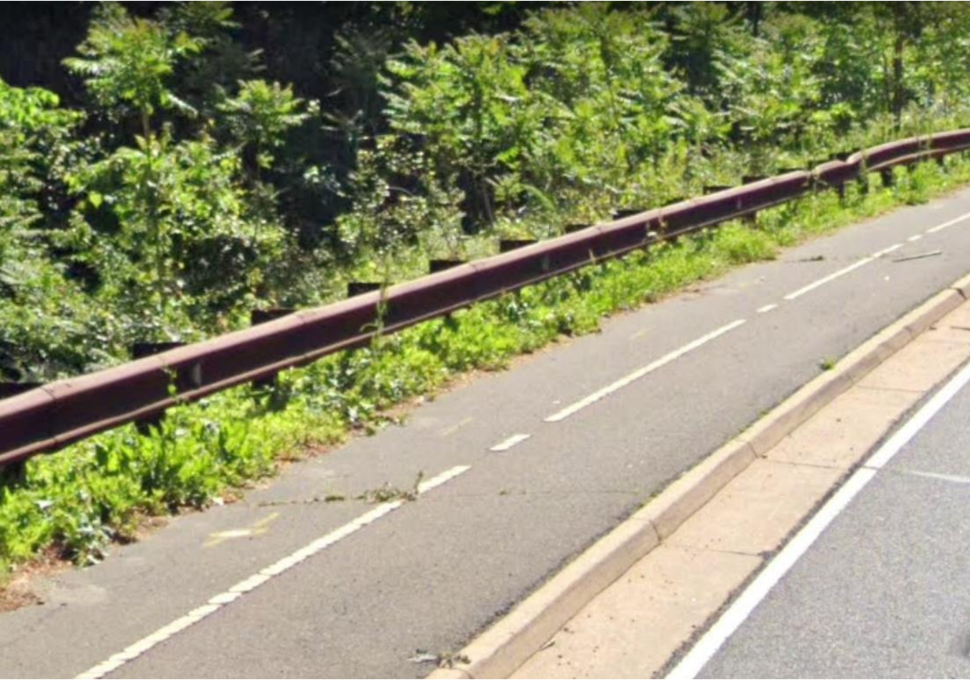
Suitland Trail with guardrail
