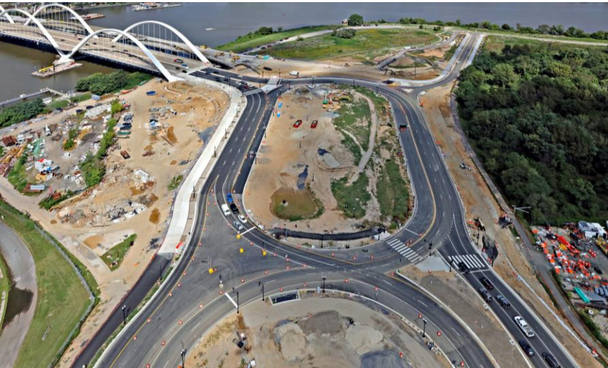
South Capitol St. / Fredrick Douglass Memorial Bridge
