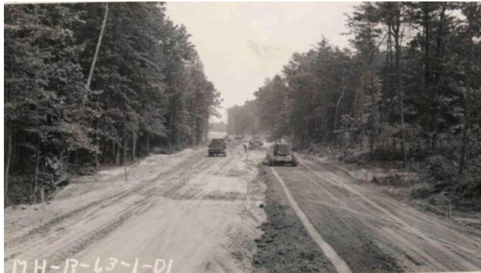
Placing Fill Material-"B" Road
