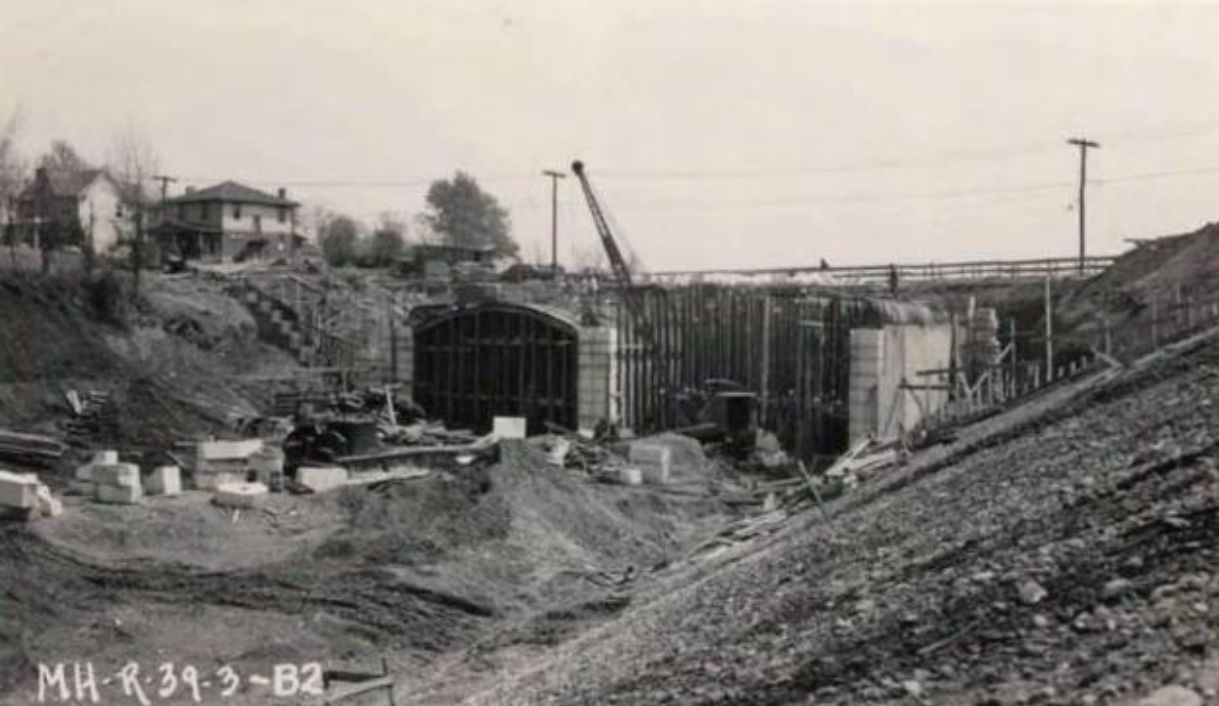
General view of west side of Alabama Avenue bridge during construction
