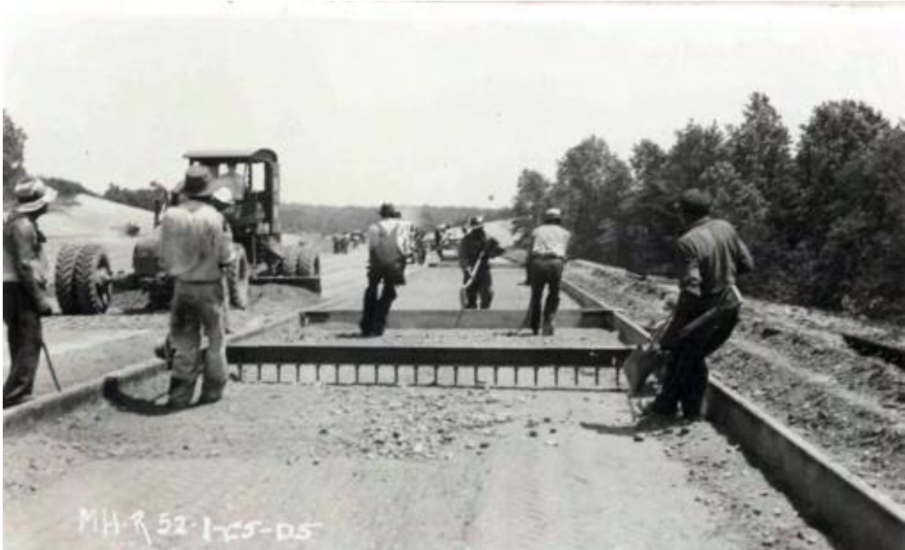
Fine Grading for Concrete Paving
